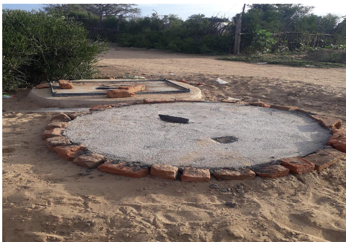
Fabrication of slabs to replace the semi-permanent plastic slabs is Section 6
